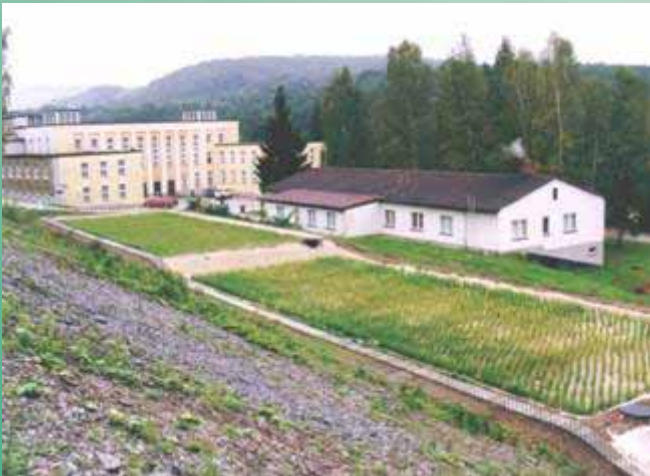
Constructed Wetland, Fa. Bioplanta
